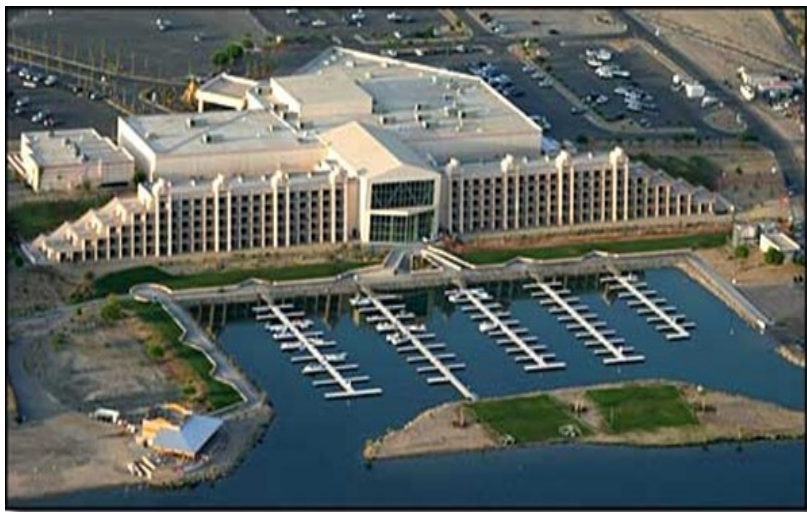
The Blue Water Resort and Casino in Parker, Arizona
